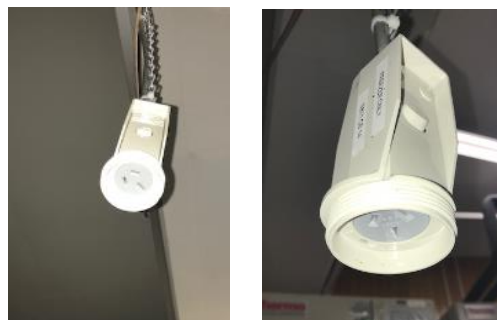
Figure 5 Suspended Pendant type - Industrial captive screw sockets – Clipsal type 56 series.
