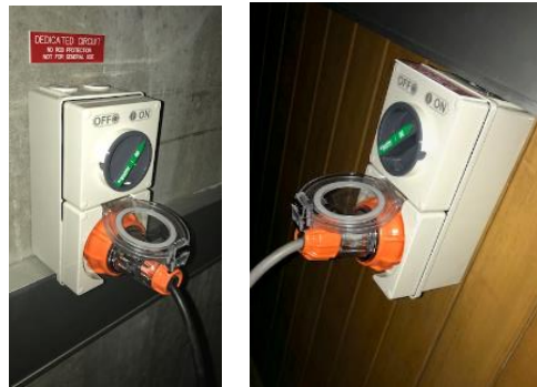
Figure 3 Industrial captive screw sockets – wall mounted- Clipsal type 56 series.
