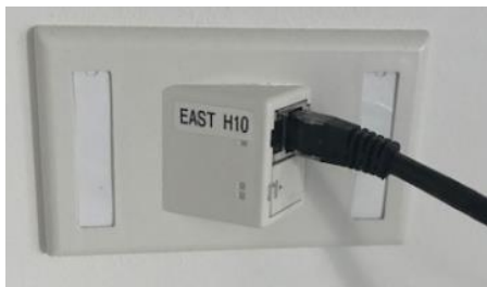
Figure 7 (a) Single RJ45 network socket.
